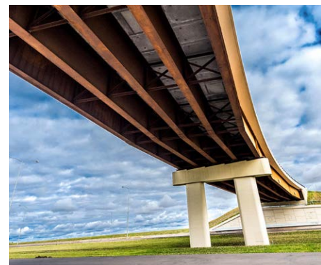
Northeast Anthony Henday Drive in Edmonton, Alberta
